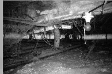
Poorly managed rainwater and warm, humid outdoor air are the two most common sources of moisture in crawlspaces.
