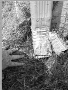
This downspout dumps rain water next to the foundation of a house – there should be an extension of the pipe to carry the water farther away from the foundation. Note also that the downspout has been crushed by people or lawnmowers.
