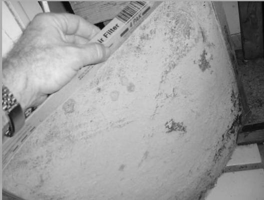
How's the filter? A clogged low efficiency filter partially sucked out of the frame.
