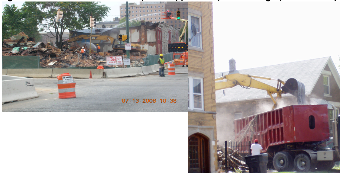
Figure 3. Demolition in Baltimore (dust suppression) and Chicago (little dust suppression)
