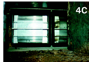
Photo 4C: Moldy air duct
