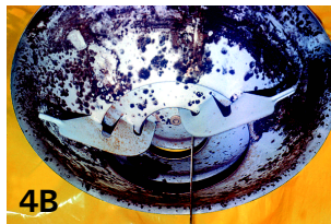
Photo 4B: Mold growth on air diffuser in ceiling
