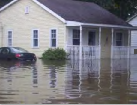
Moisture/ water intrusion
