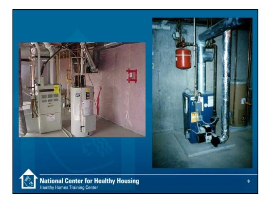
**Left picture:** A photo of a gas fired sealed combustion warm air furnace and a power vented hot water heater. A DX cooling coil has been installed in the supply side of the air handler so this is a heating and cooling system. There is no way of inspecting and cleaning this otherwise well designed system. Notice the heat recovery ventilator in the background behind the cylindrical water heater.
