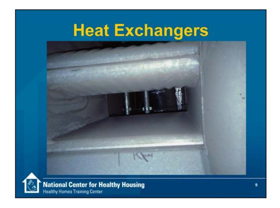
This is a photo of heat exchanger inside a furnace. We are looking at the side where inside air moved. Inside the metal tube is the flame. Two slides forward is a heat exchanger for an air conditioner.
