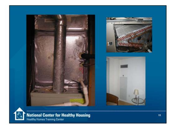
**Left:** a picture of a warm air furnace with central air conditioning. There is no way to inspect or clean the coil without opening up the ductwork.
