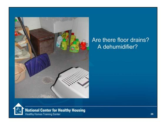
A floor drain in the basement is a good idea. It gives water from a big plumbing or rainwater leak a place to go. Notice the dehumidifier. Below grade spaces often can benefit from a dehumidifier.
