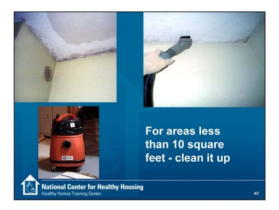
Here is a picture of mold growing on painted joint compound in a bathroom. The moisture condenses from the air during showers, in spite of a low volume of exhaust air (around 7 cfm) through the grille. The mold did not grow with one person living in the house, but began shortly after another person moved in.
