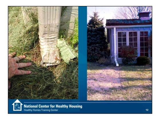
On the left is a picture of a downspout that dumps all the collected water next to the foundation. The discharge has been crushed by people or lawnmowers.
