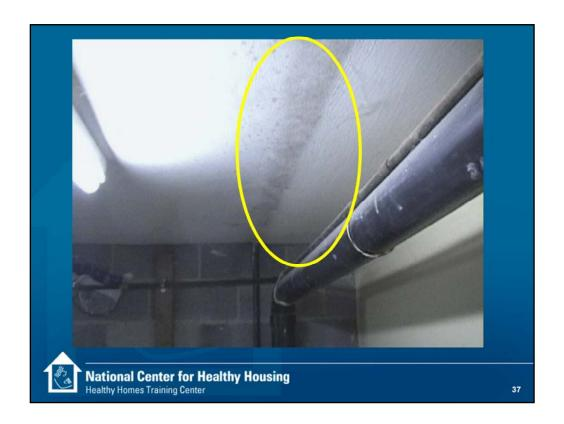
This picture shows a cold water line (seen running up the wall in the background), which condenses water above the ceiling. The water drips down onto the gypsum board ceiling resulting in a straight line of mold growth. All things being equal, mold does not grow in straight lines unless it is fed by a straight line water source.
