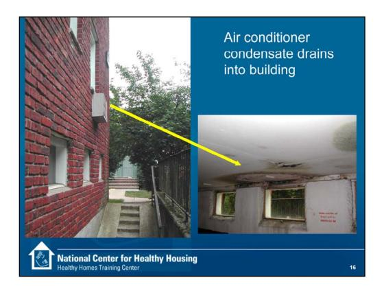
The through-the-wall air conditioner tilts towards the wall. Condensate water from the cooling coil runs into the building rather than out of the building.
