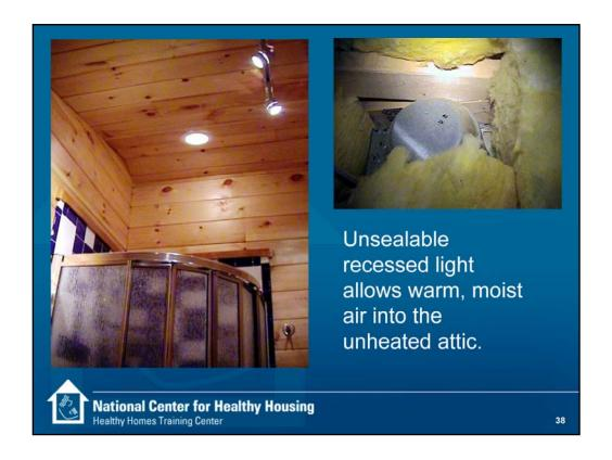
The recessed light in this photo is an opening directly into the attic. When the light is on the heat from the bulb causes a thermal draft to move even more air into the attic. This light is located over the shower in a bathroom that does not have an exhaust fan. As a result the warm, humid shower air is exhausted directly into the attic.
