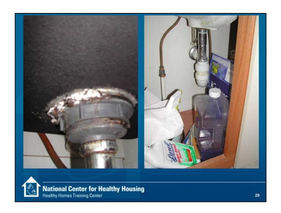
The drain basket and drain trap are vulnerable locations for leaks and vermin entry. Fortunately, they are easily inspected. Put a stopper in the sink and run water to see if the basket leaks. Let the water out to check the trap. Repair by tightening and sealing as needed.
