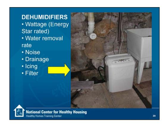
Dehumidifiers are very useful for managing humidity levels in buildings. High humidity in buildings is either the result of warm humid outdoor air entering the building or a strong source of indoor humidity. In the previous slide, the source of humidity was water migrating through the foundation and evaporating into the basement during cold weather. In warm weather, it was both the damp foundation and outdoor air.
