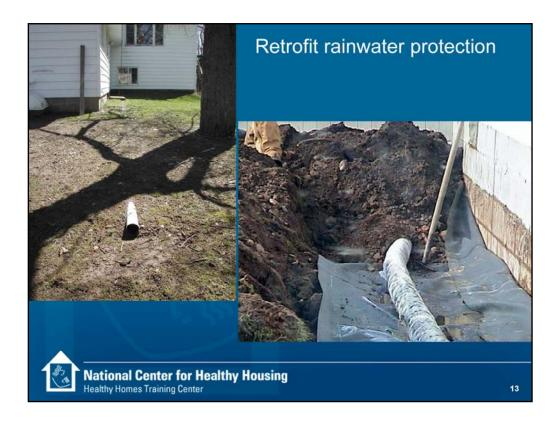
Here is a retrofit method of controlling rainwater from the exterior. EPDM rubber roofing is placed against the foundation wall and extended out below grade. Filter protected drain pipe and porous backfill are used to collect water and drain it away from the foundation. [4]
