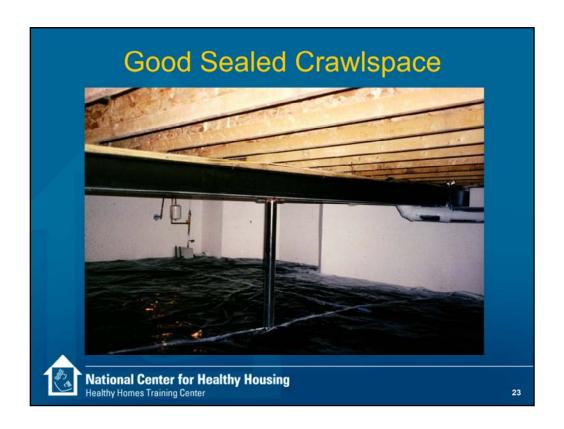
Here is a example of a sealed, insulated crawlspace with good drainage and a vapor barrier covering the soil floor.
