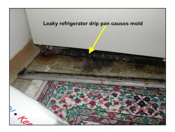
The condensation pan beneath a refrigerator may overflow and cause mold growth. Often these pans are heated to evaporate condensate. The heating may have failed. Many people do not realize they should be checked and cleaned periodically.
