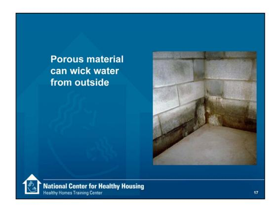
The bottom few inches of this wall are damp because water is wicking up through the footing by "capillary suction." It is only wet a few inches from the slab because the moisture evaporates into the basement. In an unfinished basement this is probably not a problem, but if the wall is finished using paper covered gypsum board, paneling and wooden studs or furring strips, a dark, damp place is created. This provides good conditions for mold growth.
