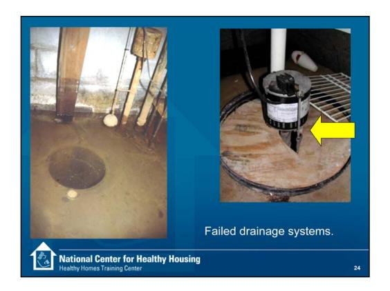
Sometimes there are drainage systems installed, but they have failed. Drain lines must be protected from clogging with silt. Traditionally they were covered with layers of straw or felt paper. In the last thirty years, synthetic filter fabrics have been developed that last longer and provide better filtration. In these photos the sump pump on the left has broken and has not been repaired. The pump on the right would run except the float that turns on the pump is stuck on the plywood cover.
