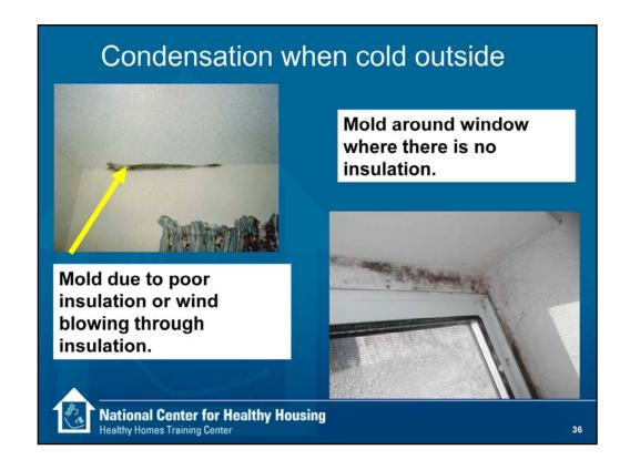
Here is mold growing on a ceiling that is chilled by wind blowing through the soffit across uninsulated gypsum board. The second picture shows mold around a window where there is poor insulation.
