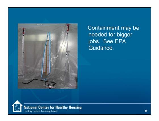
This shows fairly simple containment using spring-loaded poles and polyethylene film.
