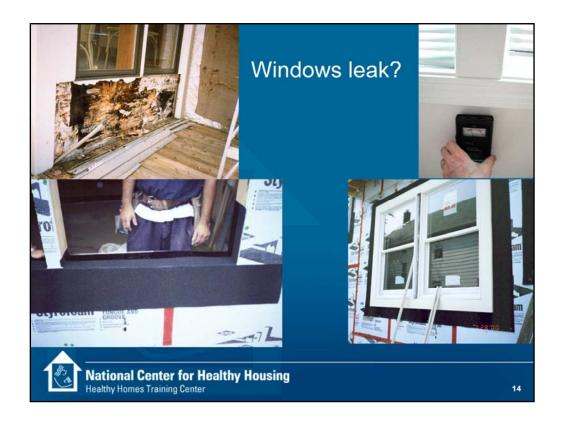
Moisture damage beneath a window. Windows may leak rainwater at mitered corners and where multiple windows are mulled together. They may leak around the edges where they should be flashed into the wall system. Use window installation methods that prevent such damage. <sup>[5]</sup>
