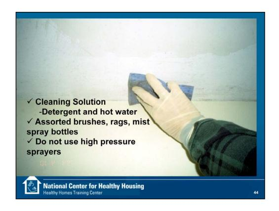
Wiping damp surfaces with water and a small amount of detergent collects any remaining fungal particles. The detergent is needed because the spores of some fungi (e.g. aspergillus and penicillium species) are hydrophobic and pushed off the surface into the air if water without a surfactant is used.
