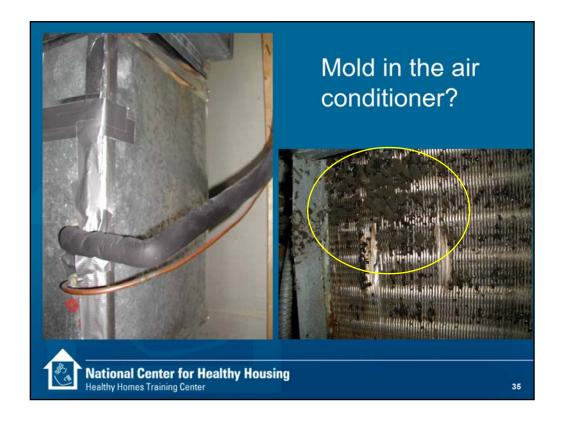
Air conditioners have cold surfaces such as the cooling coil, the drain pan, the ductwork down stream of the cooling coil and supply diffusers. Mold can grow in all of these locations. Again, there are two parts to fixing the problem. The first is to clean up the mold and the second is to fix the water issue. Cleaning up the mold should be done following guidance from EPA, NYCDOH, and NADCA. [8,9,10]
