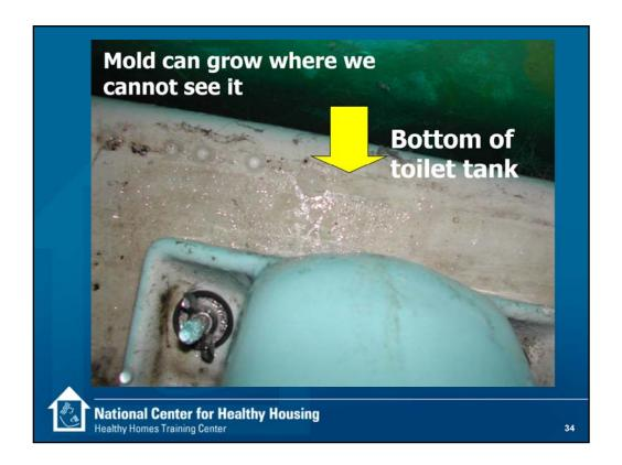
This picture shows condensation and mold growth on the bottom of a toilet tank. Condensation occurs when there is too much humidity and the surfaces are too cool. The tank is cooled by incoming cold water. The water vapor is from outdoor air during warm humid times of the year and from showers. The mold gets nutrient, not from the porcelain, but from paper dust released by tearing toilet tissue. The problem can be avoided by:
