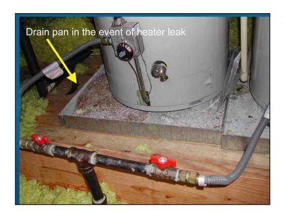
Flood pans are inexpensive ways to reduce the impact of a flood. They can be used for hot water tanks and for washing machines. But without a drain they cannot hold much. Residents need to know when there is a leak.
