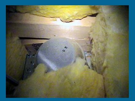
Unsealable recessed light allows warm, moist air into the unheated attic.
