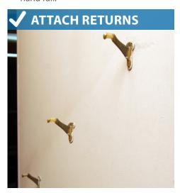
3. Mark bracket holes. Align top bracket hole with rail height mark. Repeat for top step.
