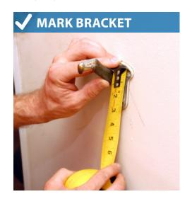
7. Measure between rail and wall. Cut return pieces to length with 45 degree angles. Attach return pieces to ends of rail with finishing nails and wood glue.
