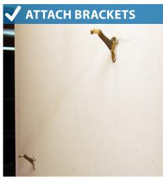
8. Attach hand rail to brackets on the wall.
