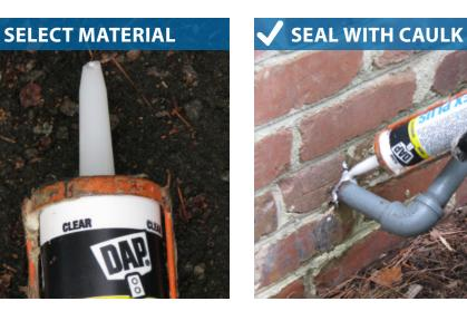
4. For holes 1/4 in. or greater, install foam backer rod and copper mesh in the hole. Seal with water-proof polyurethane or silicone caulk.
