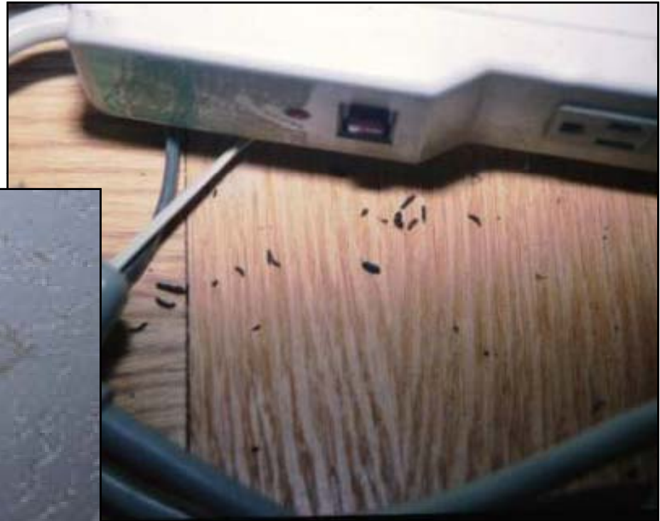
Mouse droppings by a power strip
