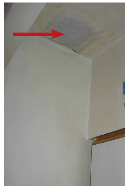
Figure 10 | Occupants blocking registers due to noise, drafts, or dirt
