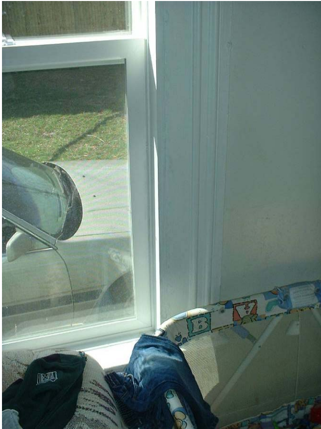
Crib next to new window
