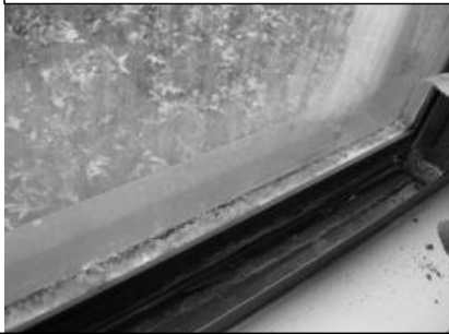
Apartment window with broken seal and unknown material settled in between panes.
