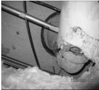
Photo taken from inside roof cavity of a roof drain. Super stated two of the drains leak within the building.
