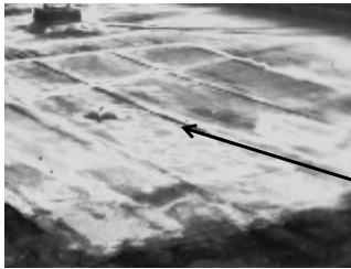
Bad roof insulation
