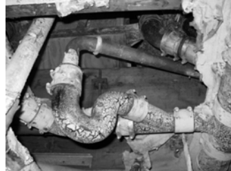
Pipe and Plumbing Chases
