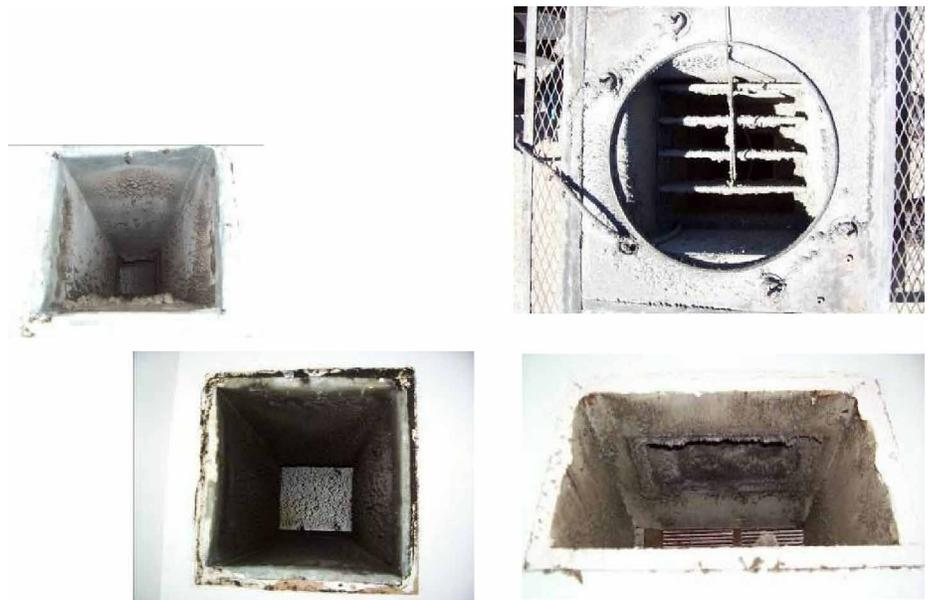
**Figure 9** | Dirt and dust clogging grills/registers and restricting airflow
