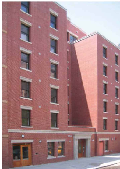
228 E 3rd Street features round metal plates visible on the exterior, which are air louvers for the individual ventilation systems in each apartment.
