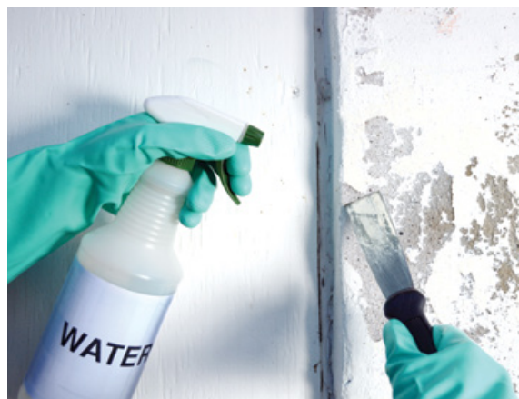
PHOTO: Wet-misting lead paint reduces dust hazard.
