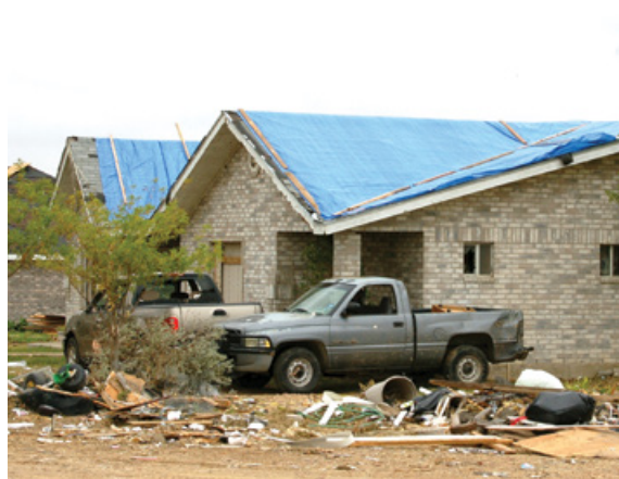
PHOTO: FEMA-provided "blue tarp" temporary roof protection.
