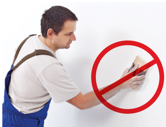
PHOTO: Do NOT sand lead paint. Use removal methods that control dust.
