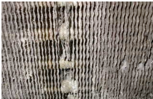
Figure 5.22 Dirty Cooling Coils Should Be Cleaned
