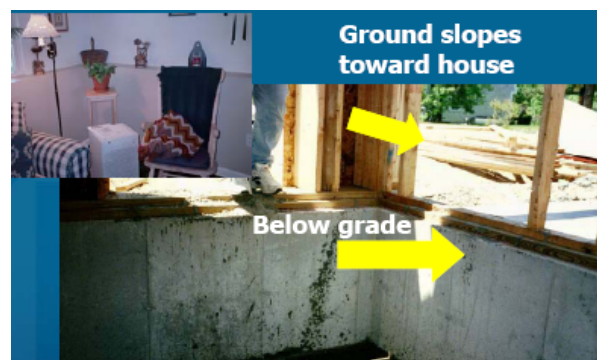
Figure 4.15 Moisture Problems Caused by Improper Ground Slopes
