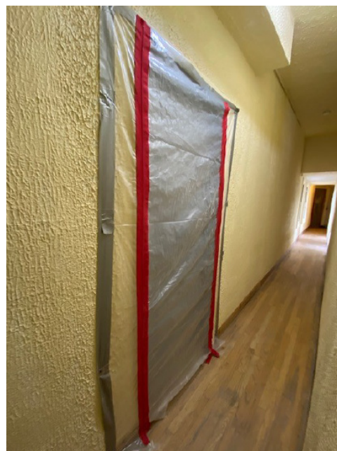
Example of a landlord-submitted photo demonstrating proper containment.
